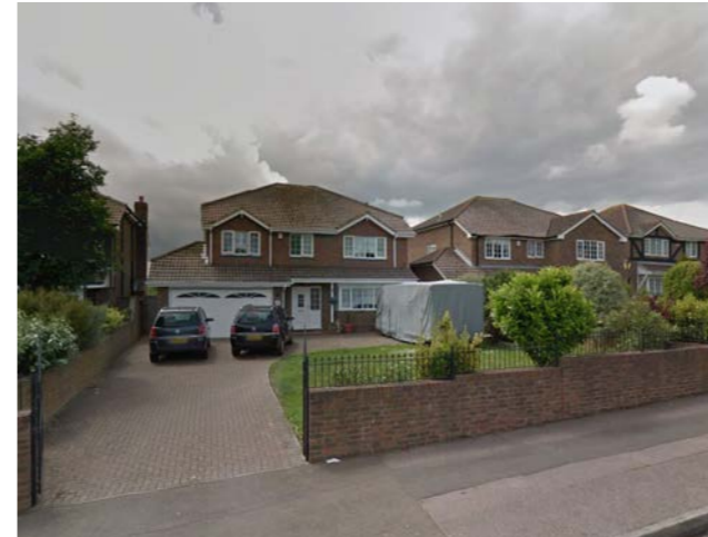
Housing on Hartsdown Road, large detached houses set back from main road.
